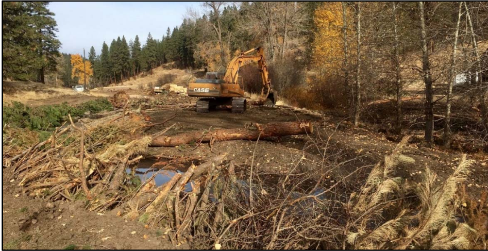
FIGURE 8 BIOENGINEERED BANK TREATMENT – WILLOW/BRUSH MATTRESS
