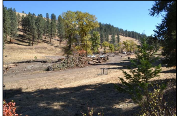
Rock Creek Construction 2018
