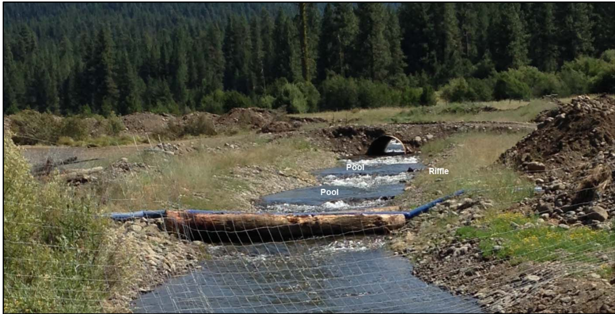
FIGURE 16 2017 TEMPORARY BYPASS CHANNEL AT MFJD OXBOW PROJECT JULY 2017. DISCHARGE OF APPROXIMATELY 35 CFS. CHANNEL SLOPE OF 2%, RIFFLE HEIGHTS OF 2-FEET. NOTE – LOG AND PIPE WERE BRIEFLY PLACED AND REMOVED.
