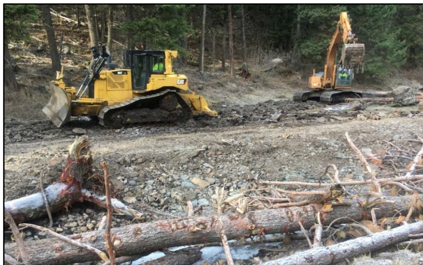
FIGURE 9 DRAW-BOTTOM ROAD DECOMMISSIONING
